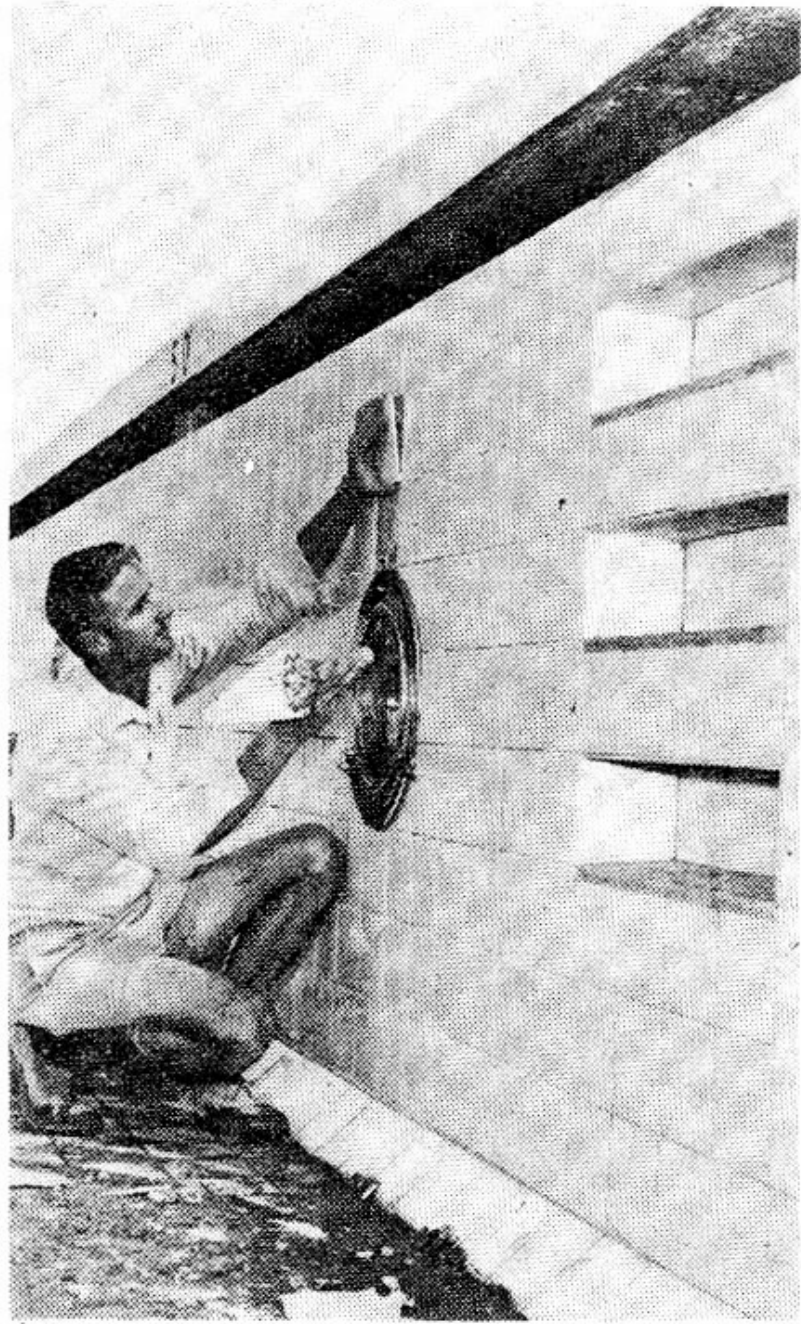
BELOW: A tiler at work.
